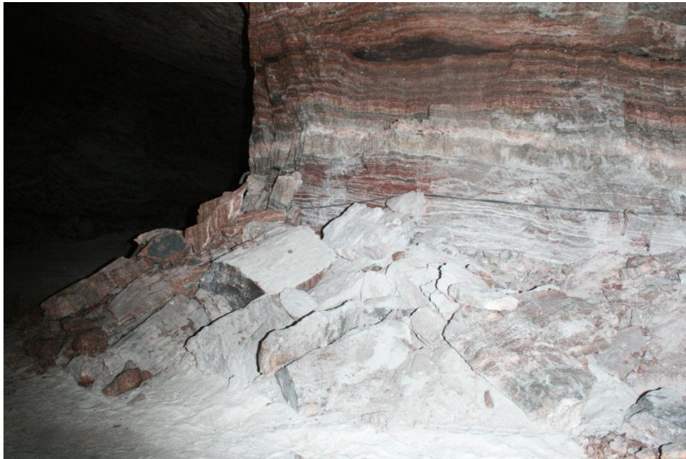
Figure 6: signal cable with salt cover after (natural) fall of salt on the cover
