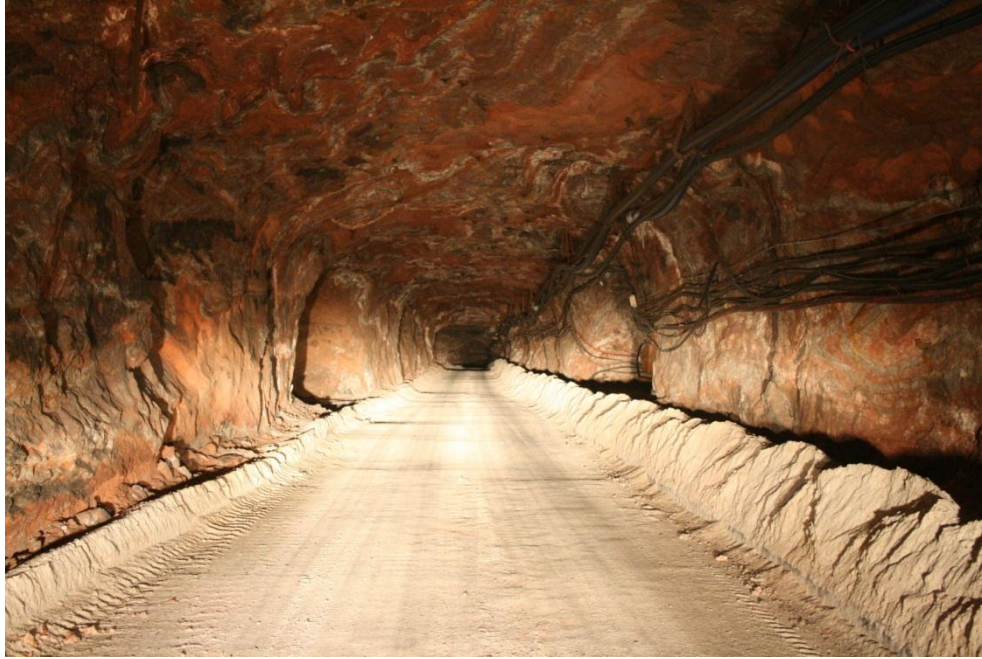
Figure 5: signal cable with salt cover
