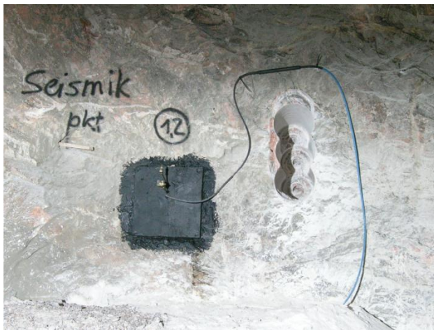
Figure 4: scheme of installation of the seismometer in a pillar and after installation cable and cable ways
